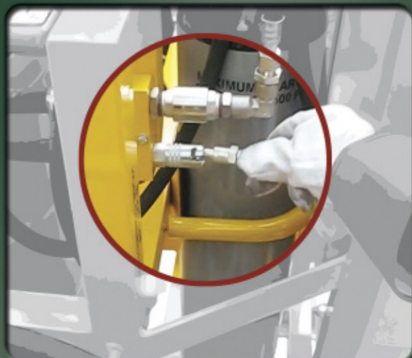
Connect blow-off hose to rig's nitrogen supply
